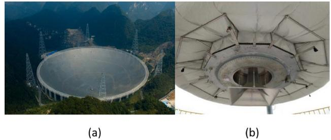
**Figure 1.** A picture of FAST (a), equipped with the ultra-wideband (UWB) receiver (b).
